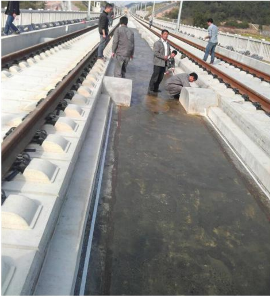
图四：沪昆高铁杭长线高铁防水涂料底漆涂布
